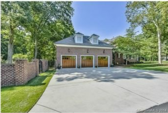
Unrivaled attention to every detail. Brick 2.5 story located in the heart of Foxcroft, a signature neighborhood. .73 acre lot. 3 stairways, Family room opens to kitchen. Finished 3rd level. Main level
